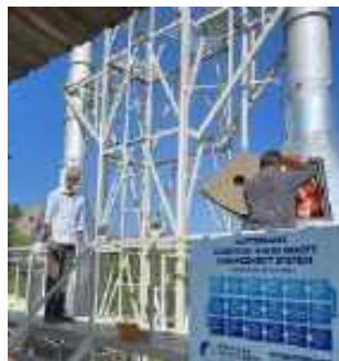
New incinerator to improve processing capacity.
